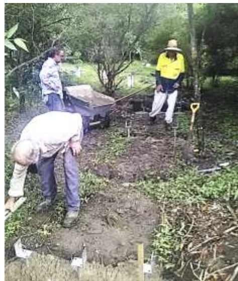
Don, Michael and John putting in foundations of a small walkway over a boggy area in Room 5 early this month
